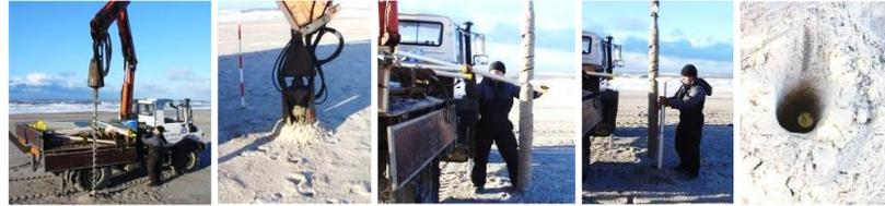
The PEMs are placed 1-3 ft. below the beach surface, making the entire installation invisible to the naked eye. The PEMs are not connected and no energy is used to operate the system.
